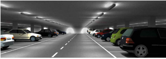
Standard position: the power output of the luminaires is dimmed to 10%, thus obtaining a minimum level of lighting.
