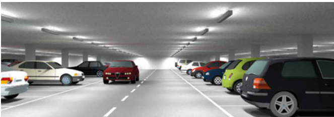
As soon as the luminaires detect the presence of persons, or the level of natural light falls below a minimum set threshold, the CF function is activated and they switch to 100% power output for the set duration (this can be regulated during installation).
